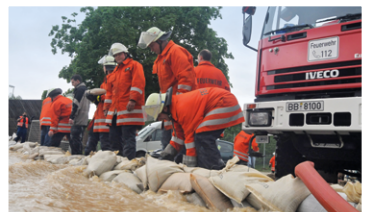
Protective walls of sandbags
